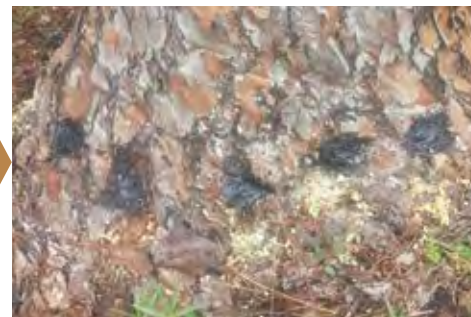
Fig. 4: Roofing tar was used to cover the holes.
